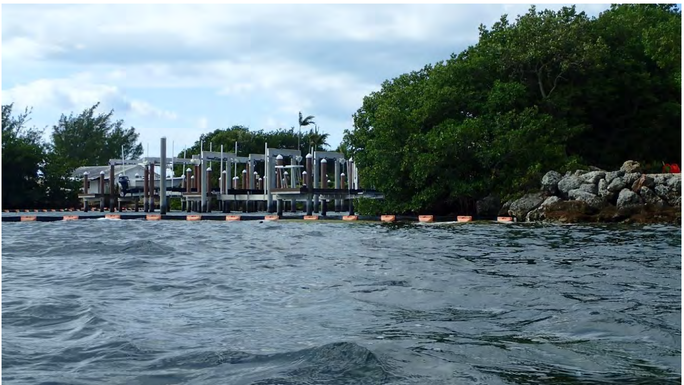
Photo of existing dock structures within the boat basin.
